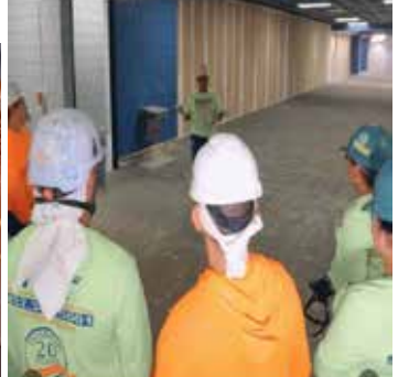
WE OFFER STRUCTURAL DEMOLITION ON TIME AND ON BUDGET
